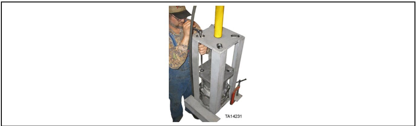
Figure 97: Installation of bolts securing outer housing
