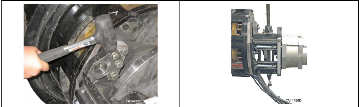
Figure 44: Tapping on torque tube to ensure it is not in a bind prior to adjustment and positioning of pipe clamp for adjustment of torque tube
